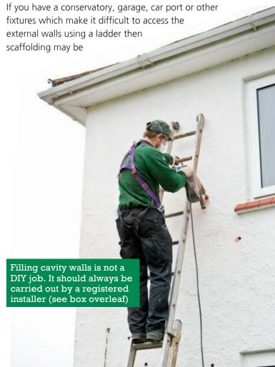
required and this will add to the cost of the work. Some installers make use of a telescopic lance system for hard to access walls. Using the lance the insulation material is injected by entering the cavity end-on, rather than drilling through into the cavity at 90 degrees. With new-build properties rigid insulation boards are often fitted into the cavities as part of the construction process.
